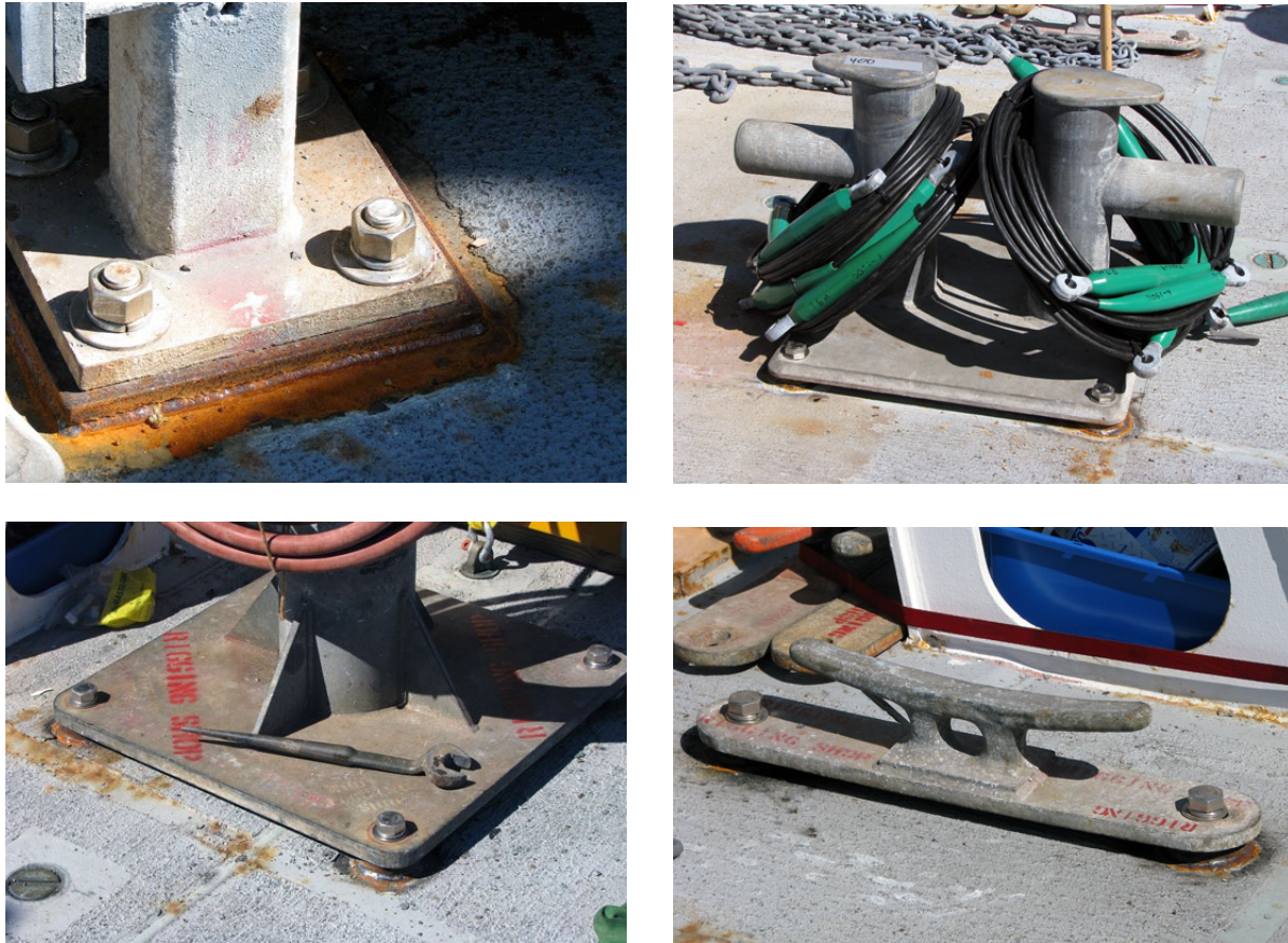
Fig 4-3: Examples of deck welding necessary to accommodate mooring deployment gear on the deck of the Hi'ialakai . Square plates with bolts extending vertically were used for the TSE winch (upper left) while threaded disks were used for the H-bit, cleats and air tuggers (clockwise from upper right).
